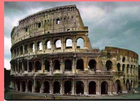
**Coliseum** - The Coliseum consists of four floors: the first three of them have 80 holes shaped like archs, while the fourth is taller than the others and is characterized by a more compact building mass with windows. The archs are separated by pillars with semi-columns of Doric, Ionic and Corinthian order. It is the greatest amphitheater of the Roman world.
